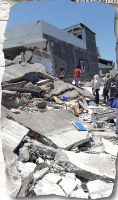
帕魯堂倒塌損毀
